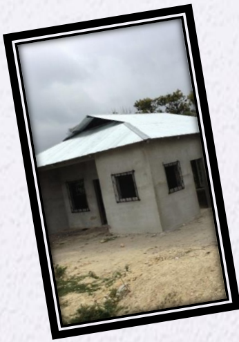
Construction begins on the first free-standing Birthing Center in the Petén.
